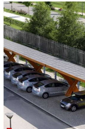
Power electronics Energy management
